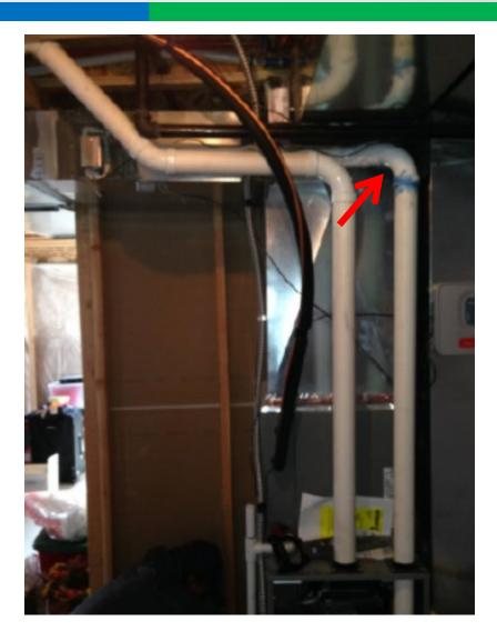
Horizontal sections less than 4 feet must have a minimum <sup>1</sup>/<sub>4</sub>" per foot slope to the furnace.
