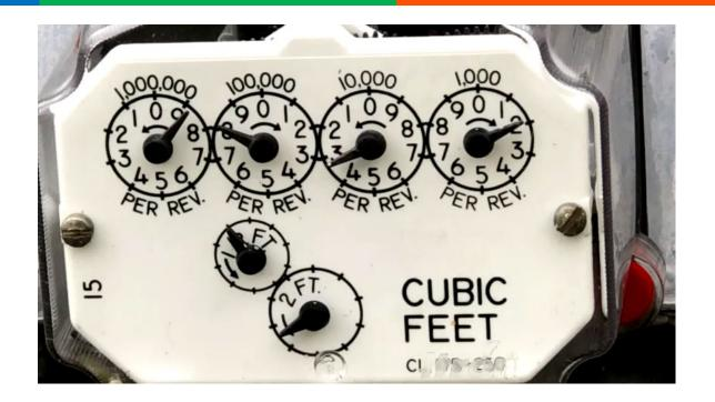
We clocked the meter, and it takes 32 seconds to consume 1 cubic foot of gas
