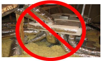
Utilizing proper ductwork design and installation methods is crucial to ensuring that the system is delivering the correct airflow and space conditioning. Poorly design duct systems result in less efficient systems, customer complaints, and reduced system longevity.
